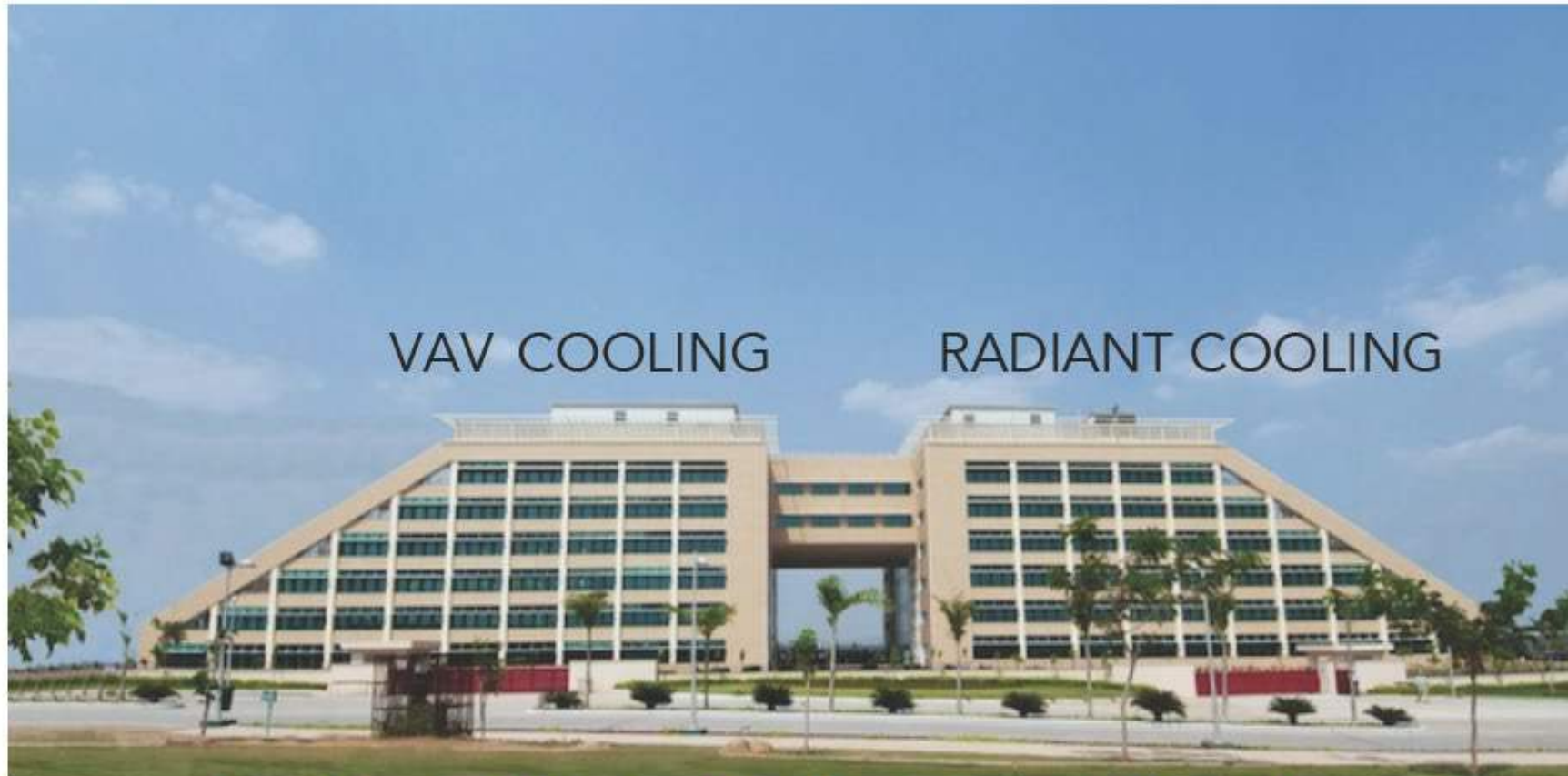
Figure 1 - Infosys SDB-1 Hyderabad - 125,000 sf of radiant cooling and 125,000 sf of VAV cooling
