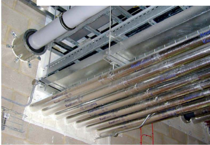
Figure 5.12 Professional and nicely performed firestop of penetrations Model of cable transit systems
