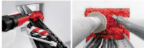
Figure 5.10. Two pictures with examples of expanding firestop foam
